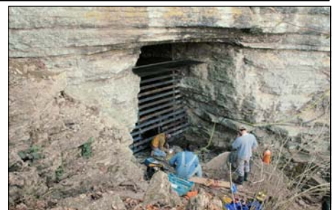
Building the gate. © Cory Holliday/TNC
